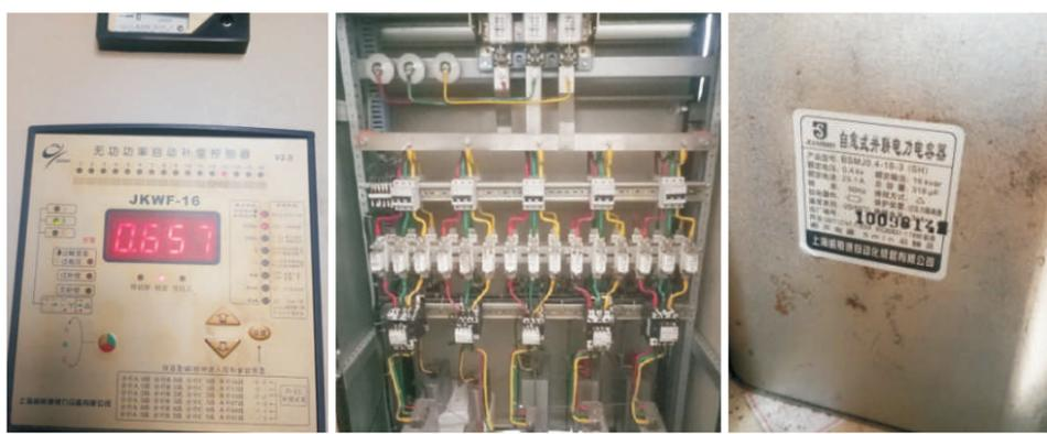
Fig\_5 Reactive power compensation equipment
